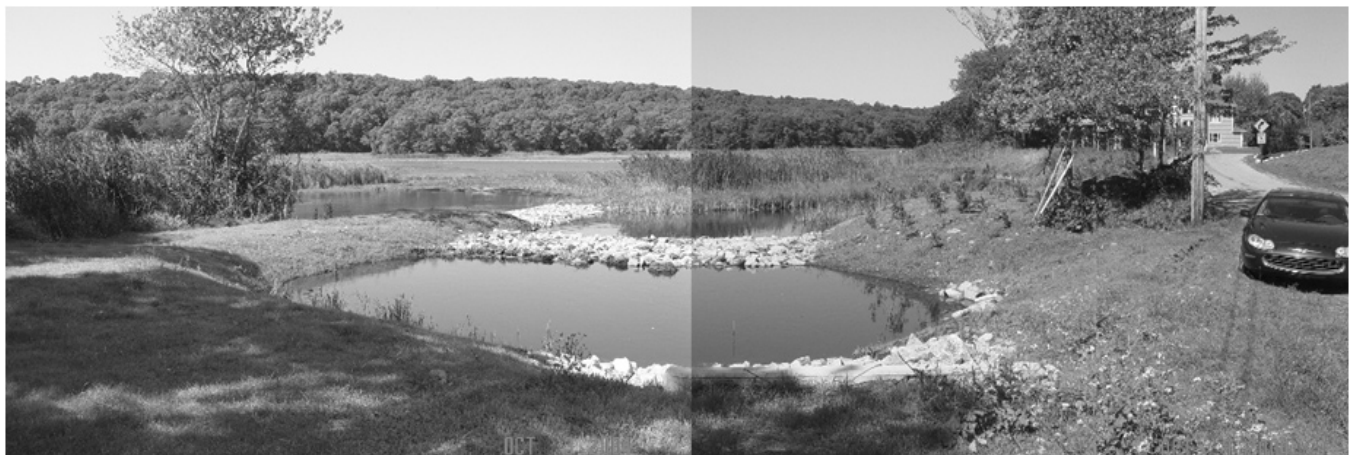
Circuit Drive Detention Pond System
