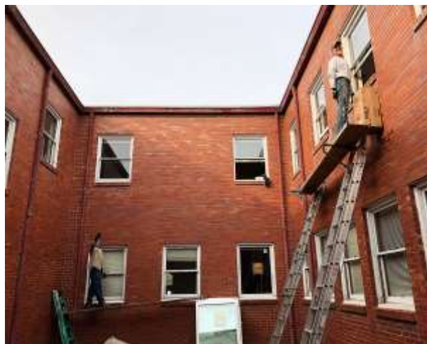
Sun Windows' is doing an excellent job on the installation. What a difference a window can make!
